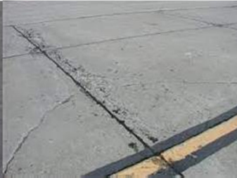
Figure 3.3: Heavy scaling
