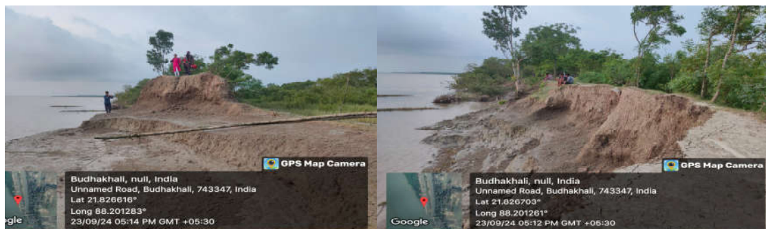
Fig-3: River Bank Erosion
