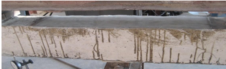
Figure 3.36 Top FRP of Beam TB1 before Testing
