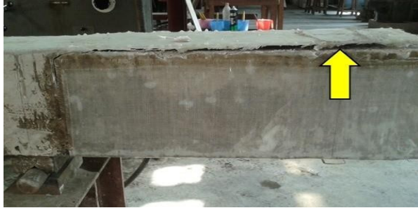
Figure 3.19 U-jacketed GFRP wrapped on the Beam SB3
